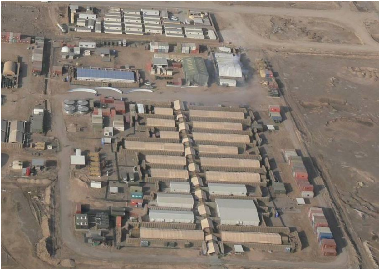
Tier 2 Hospital accommodation at the Contingency Operating Base, Basrah Air Station (Note blast walls around hospital departments for protection against indirect fire)
