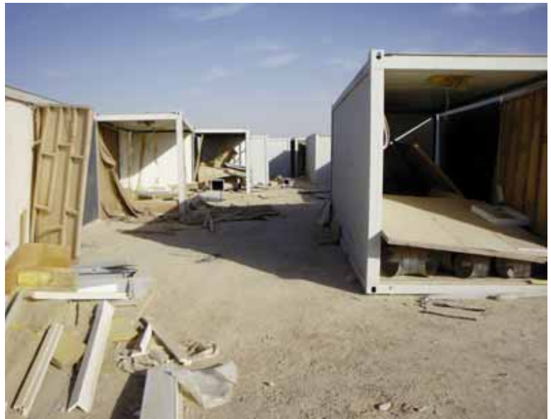
Figure 2. Basra Hospital having been relocated to a BSN compound.
