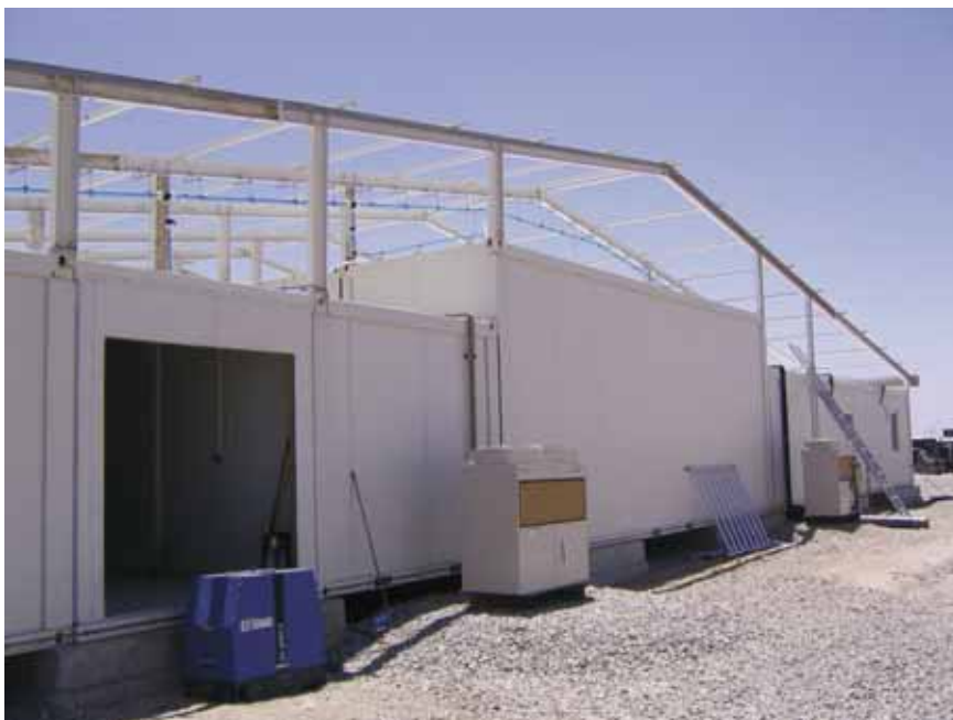
Figure 6. Steel frame cabins clipped together.
