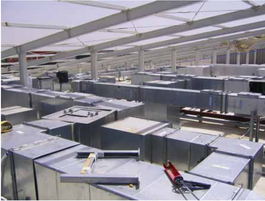
Figure 7. The roof void with services under construction.
