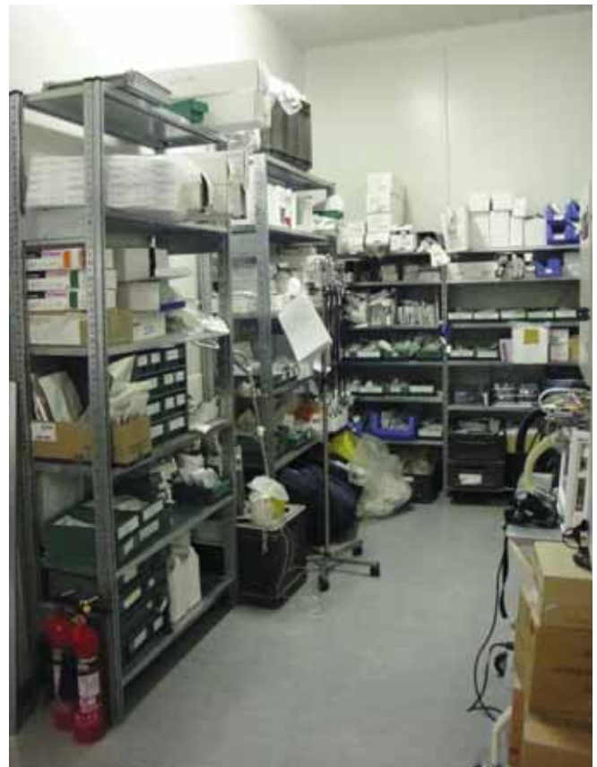
Figure 10. Corridor outside operating theatre crammed with storage blocking bed egress.
